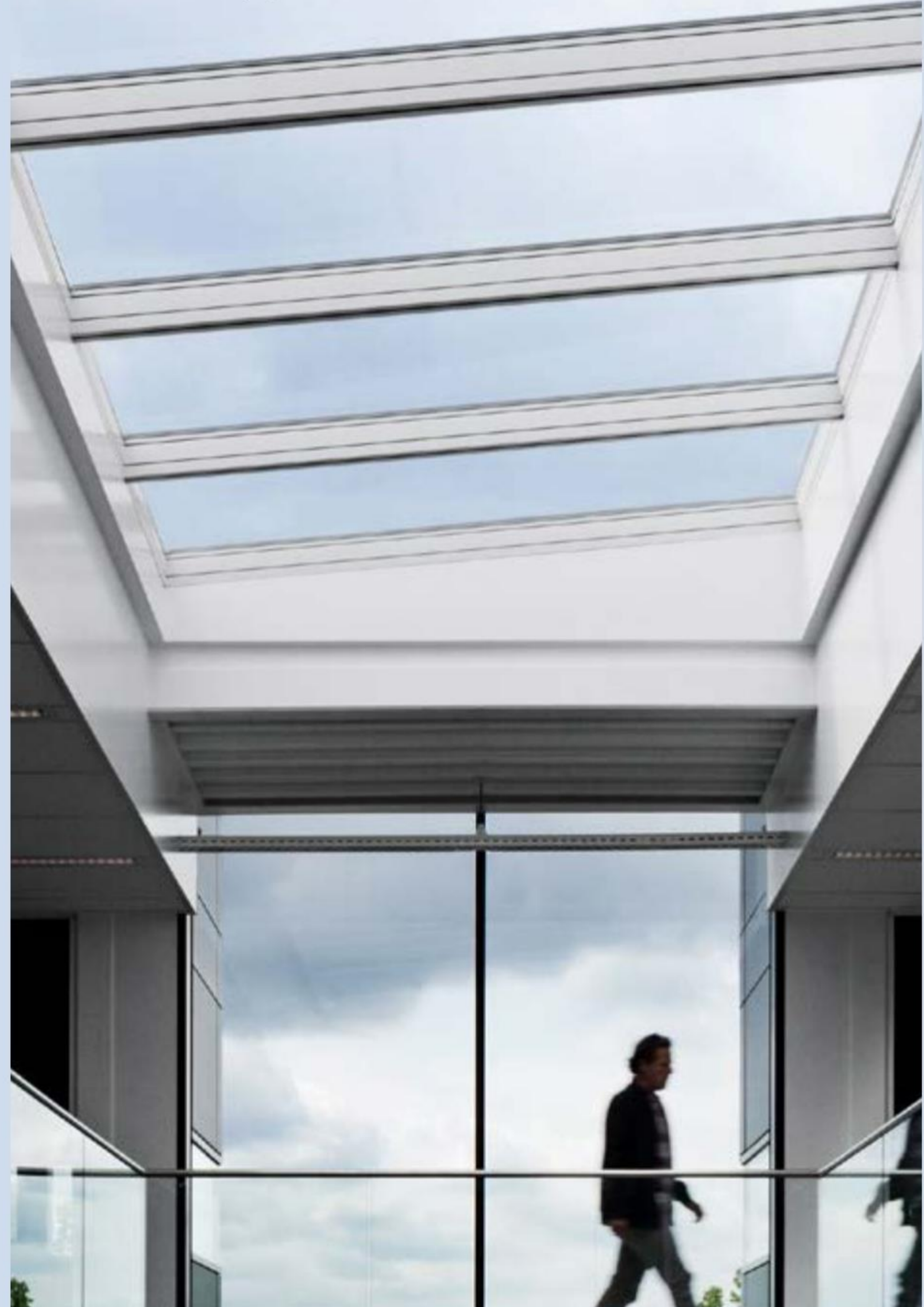
VELUX Modular Skylights in offices in Vordingborg. Photo: VELUX A/S, 2013.
